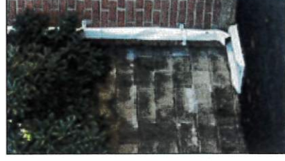
Downspouts for roof runoff
